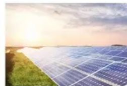
Energy Storage System
